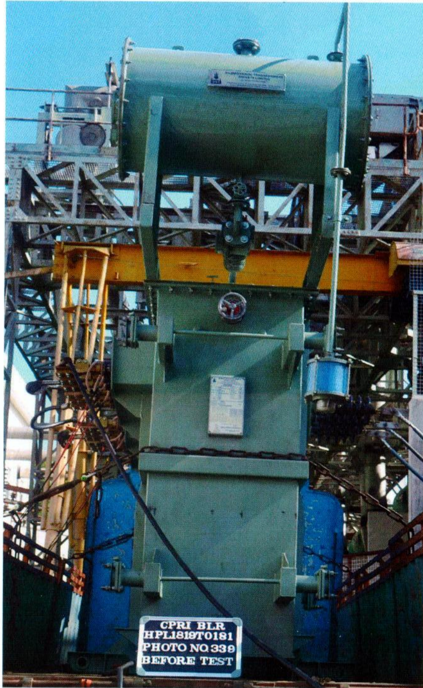
Photograph No. 339: Mounting arrangement before short-circuit test
